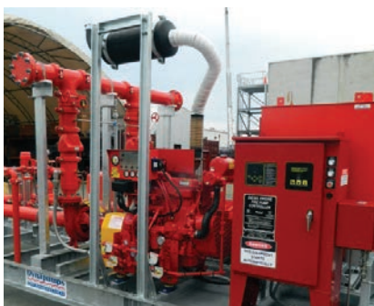
Large package firepump set built in Western Australia
